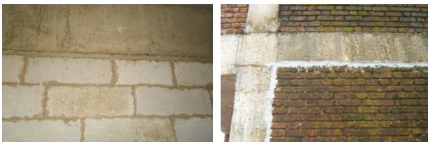
Between RCC & Wall-top layer
